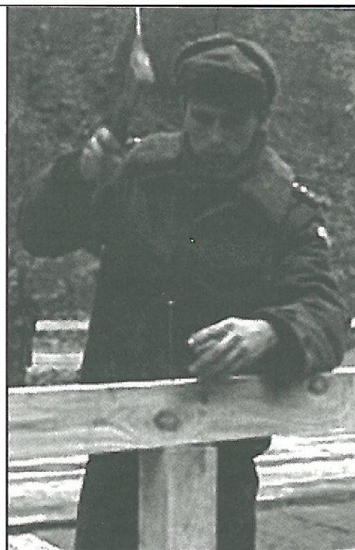
A Hungarian engineer works on the bridge at Basci.
